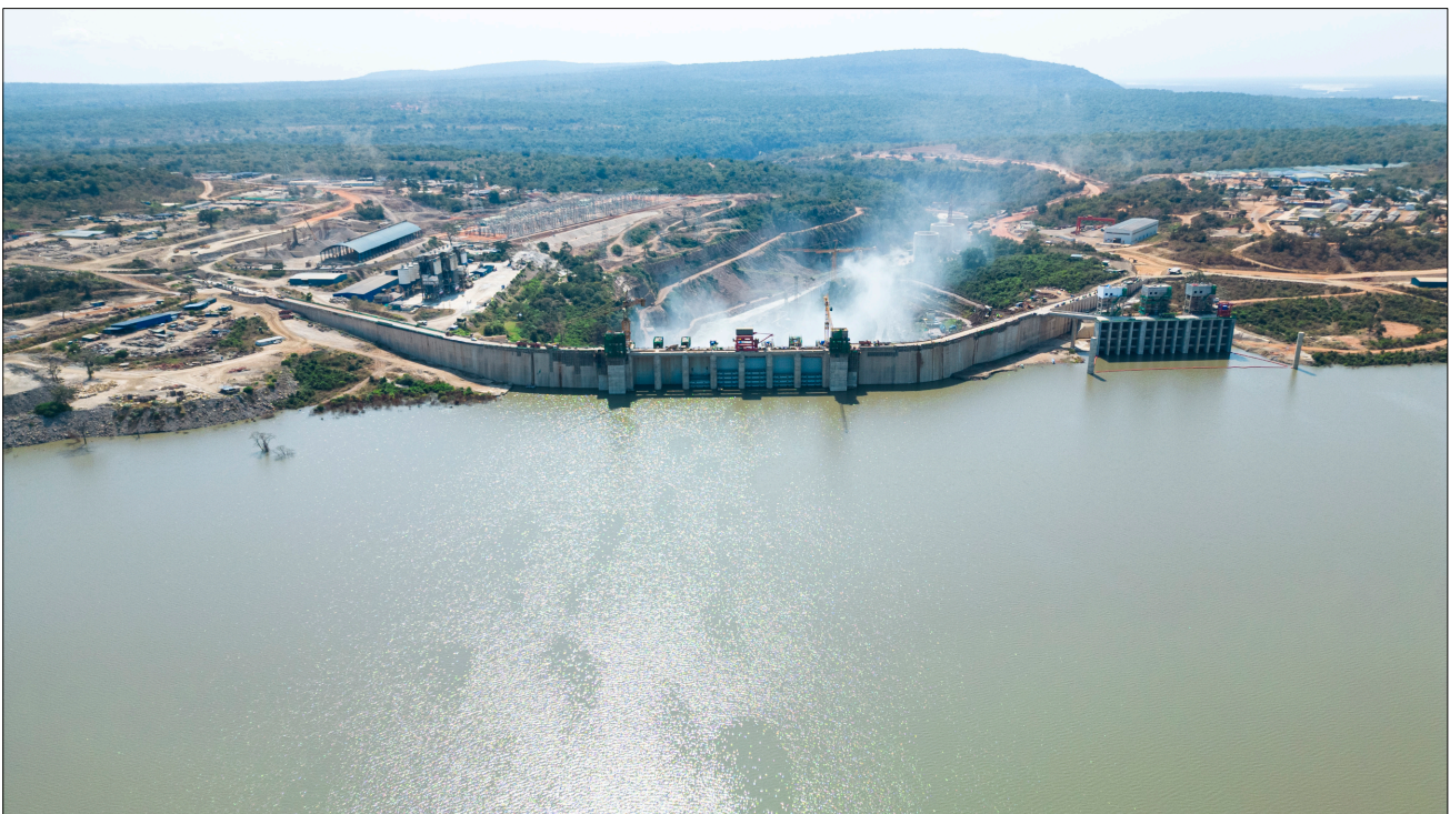
The Julius Nyerere Dam in Tanzania. (Picture Elsewedy Electric)
