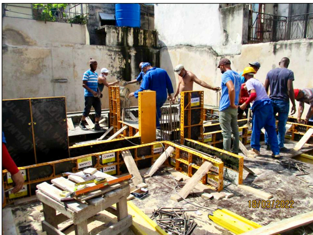
Construction site in Old Havana. (Picture ma)
